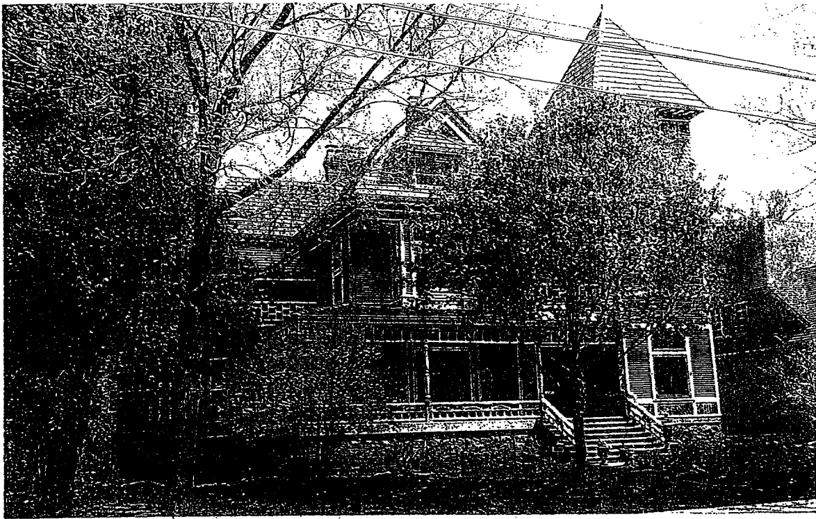
The Philo W. Stacy House 677 Highland Avenue, Glen Ellyn Spring, 2005 Front (west) Elevation
