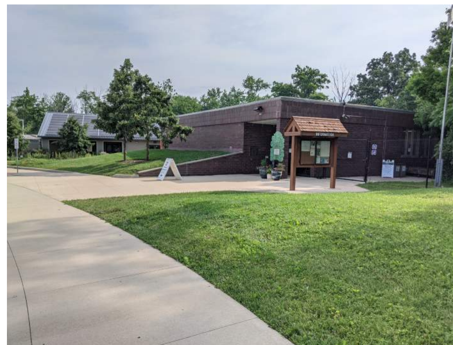
PHOTO 3 - EXISTING CLINIC BUILDING
