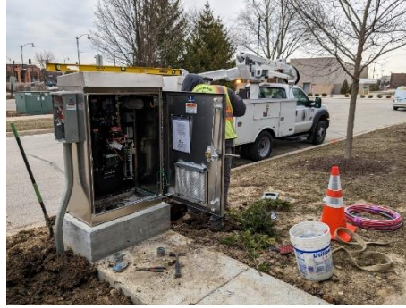
Street Light Controller Installation on Taft Avenue
