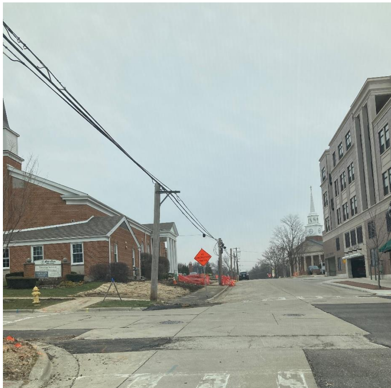
Hillside Avenue Utility Undergrounding Facing west on Hillside Avenue at Main Street Note, Tops of Poles Cut Off With ComEd Facilities Removed
