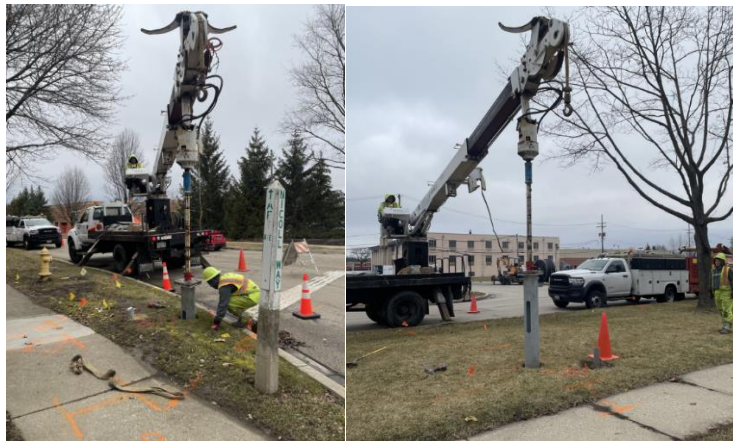
Street Light Foundation Installation on Taft Avenue
