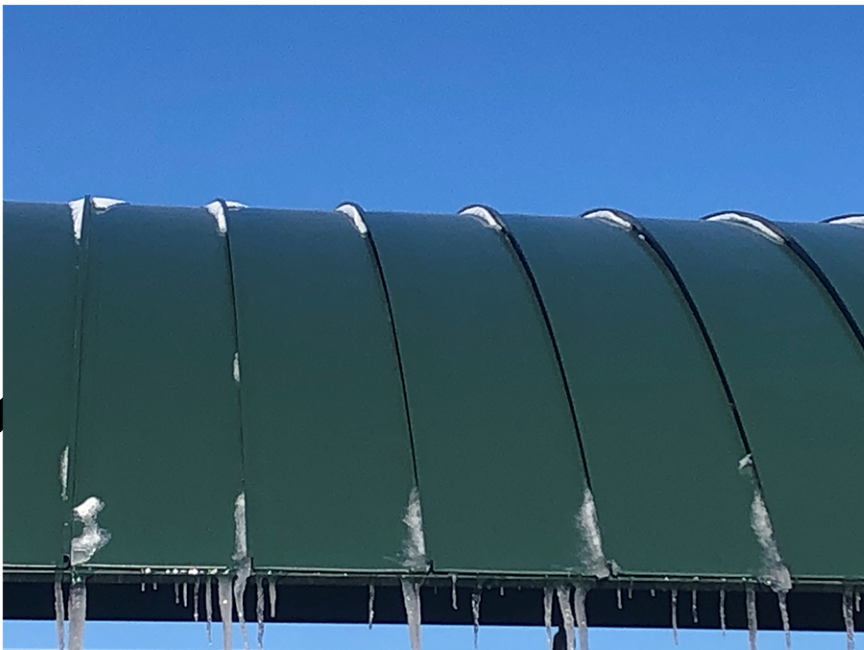
PREFINISHED STANDING SEAM METAL ROOF 'FOREST GREEN'
