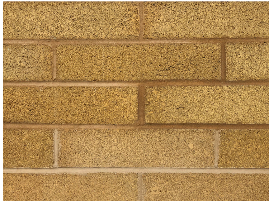
UTILITY BRICK VENEER 'BUFF' TRASH ENCLOSURE (NOT SHOWN IN PICTURE)
