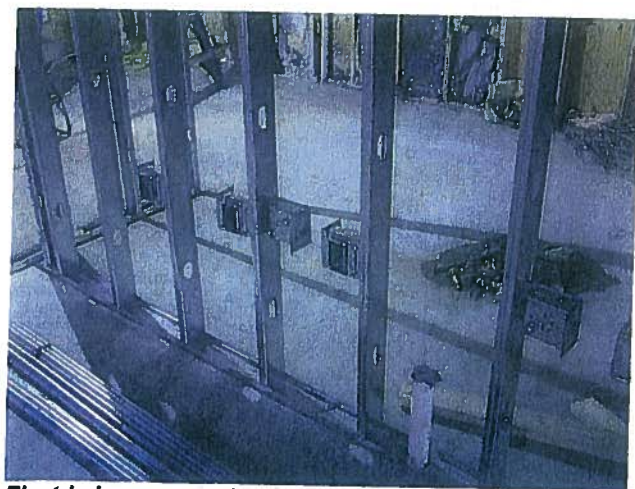
Electric boxes were installed in the kitchen.
