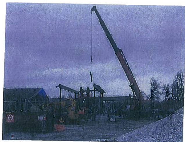
The circle drive main canopy came together quickly.
