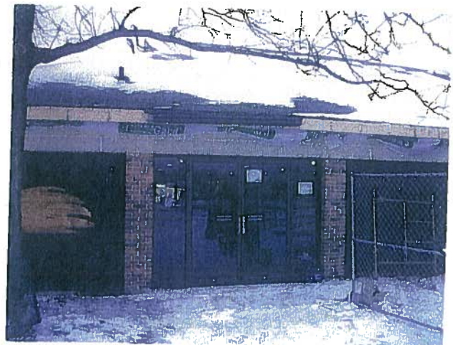
The sand colored Frieze Board has been installed over the east Pro Shop doors. The Frieze Board will protect the wood from water damage and give the building a new look.
