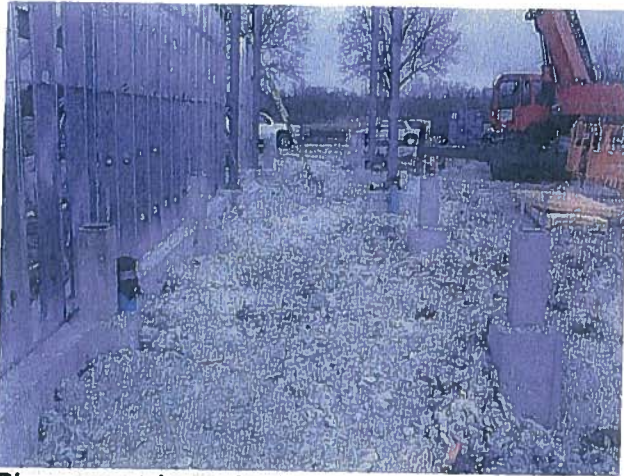
Blue-green stubs are in place where the downspouts will connect to drain pipes below. It was too cold for the excavator to work on the downspouts on the west side of the building.
