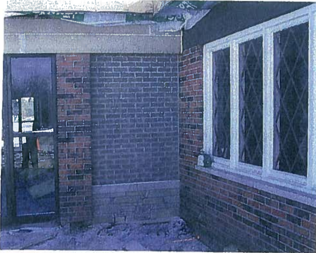
The masonry sample wall - brown brick above a limestone capped course of stacked stone - met with the architect's approval. The original red brick will be stained to match the new brick.
