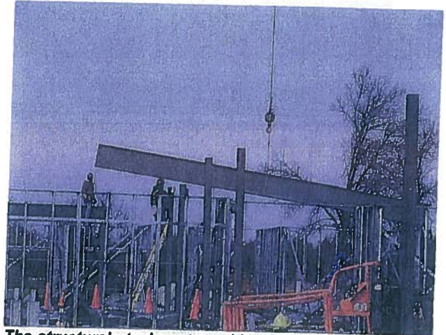
The structural steel posts and beams were installed at the end of the week, when temperatures moderated a bit.
