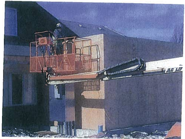
The carpenters began sheathing the exterior walls with plywood. This is an example of work being done out of sequence due to the delay in delivery of the roof trusses.
