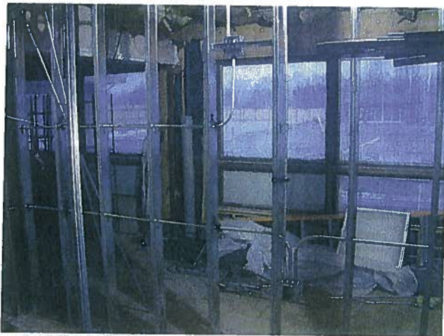
Work continued in the kitchen. Electric conduit was installed to connect the outlet boxes installed last week.
