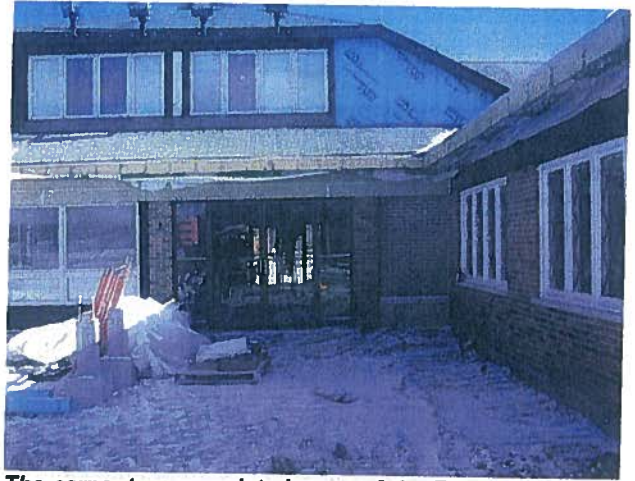
The carpenters completed more of the Frieze Board installation over the West Hallway Entrance Doors.
