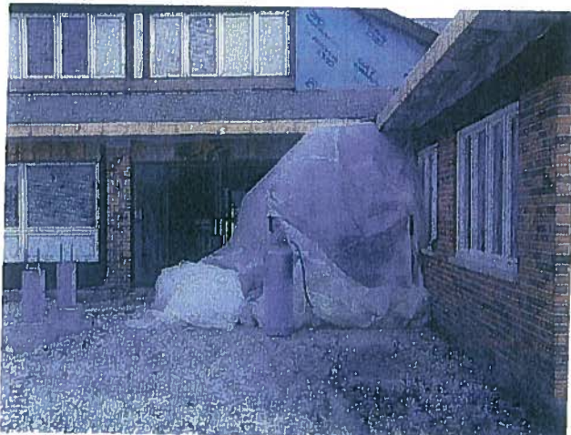
A mason was on site this week to build a sample wall of brick and stone work. He did his work under a tarp, to keep it from freezing until the cement had cured.
