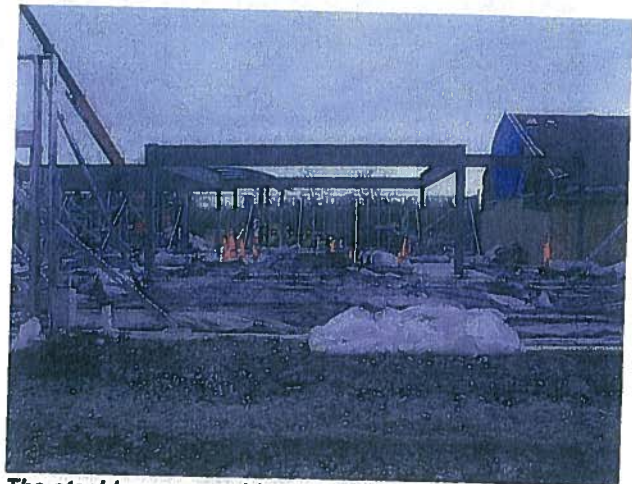
The steel beams provide the base on which the roof trusses will sit.
