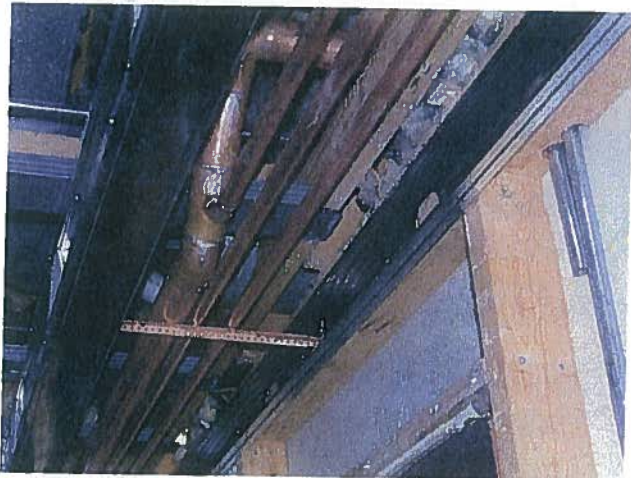
The water pipes are being run in a ceiling soffit to prevent them from freezing. The addition of that soffit in the kitchen eliminates the need for extraordinary pipe insulation and greatly reduces the risk of pipe breakage.
