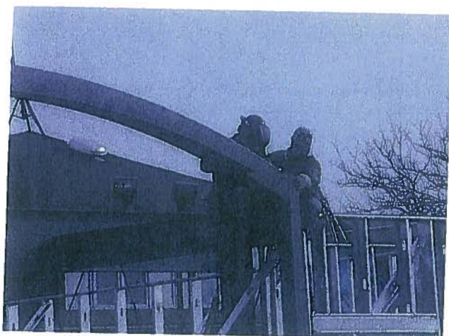
The Iron workers were on the site for three days, finishing with a rare workday on Saturday.
