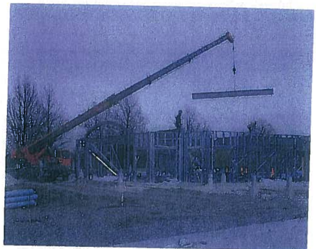
It only took one day to put all of the steel beams in place.
