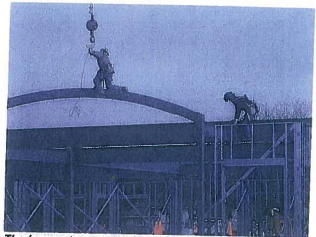
The banquet room arched beam is unhooked after being set in place.
