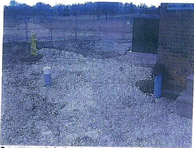
Down spout drain lines are complete on the east side of the clubhouse.
