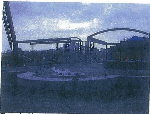
The arched barrel vault and the arched main canopy are key elements of the clubhouse addition.
