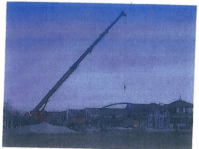
The crane sets the barrel vault beam for the banquet room on the west side of the clubhouse.
