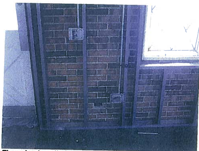
They also installed electrical outlet and switch boxes in the meeting room. Earlier in the week the carpenters completed framing the new walls in the meeting room.
