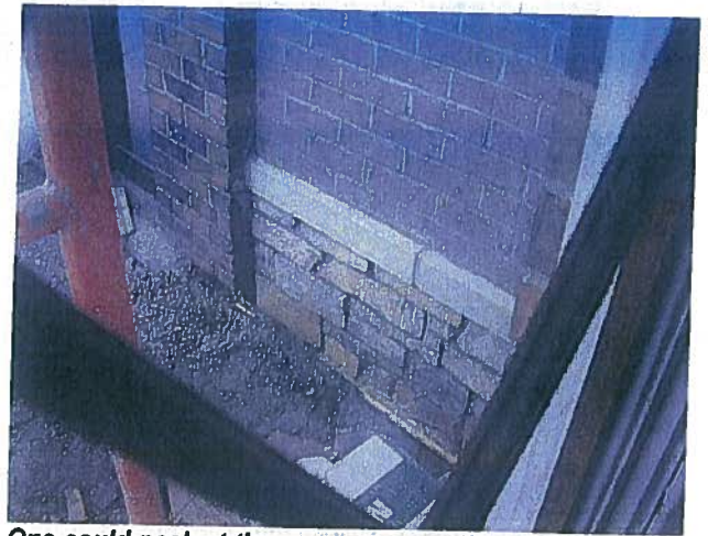
One could peek at the masonry sample wall that included a stacked stone base, a stone cap, with face brick above.
