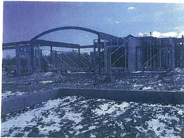
The installation of plywood sheathing has just started. The sheathing will provide workers some protection from the elements and will make them more productive.
