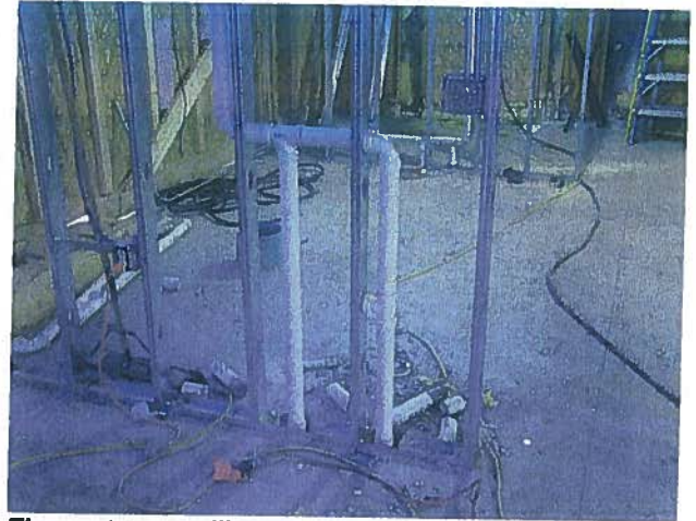
The contractor will provide connection points for water, sewer and electric. Village Links staff will install most of the kitchen equipment.
