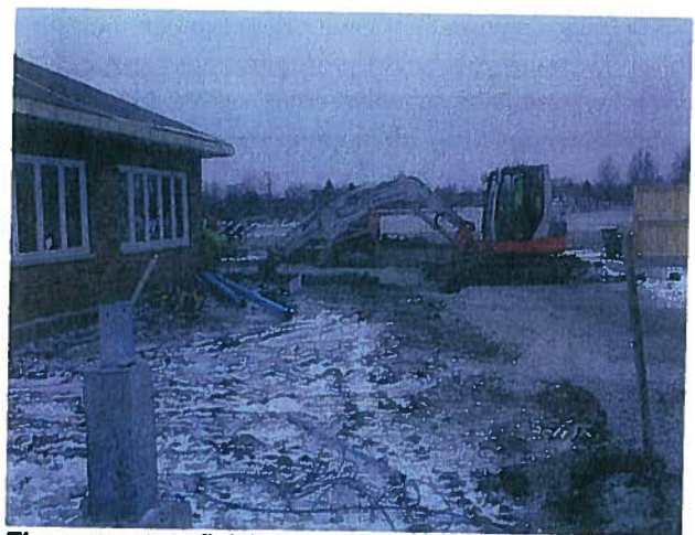
The excavators finished the installation of below ground down spout drains on the west side of the clubhouse.
