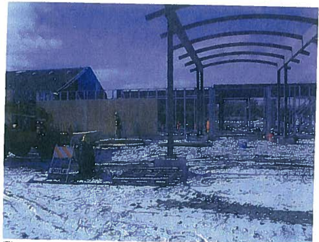
The plywood sheathing could not be applied until the structural steel was in place. The structural steel gives the walls enough support so they will not be blown down by heavy winds.
