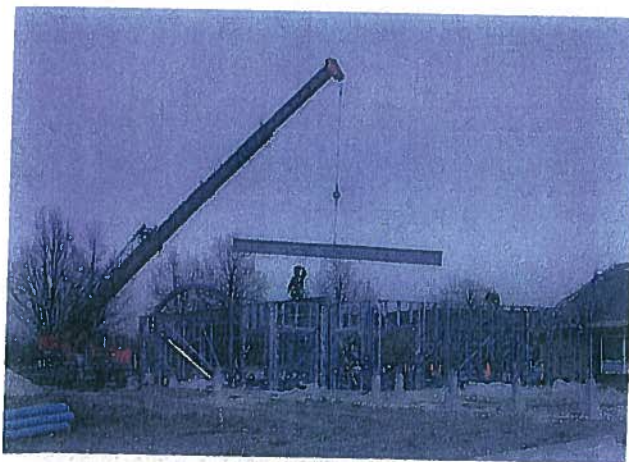
Iron workers set the steel beams loosely in place, and went back later to connect the beams with bolts and welds.
