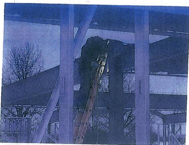
Iron workers bolted and welded the steel beams together.
