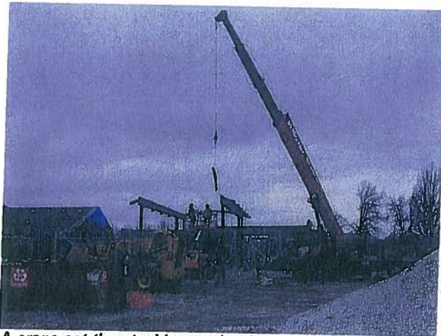
A crane set the steel beams in place.
