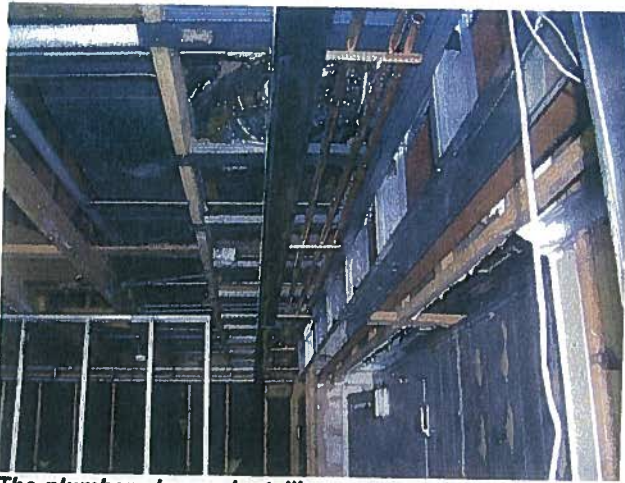
The plumbers began installing copper water pipes overhead in the kitchen.
