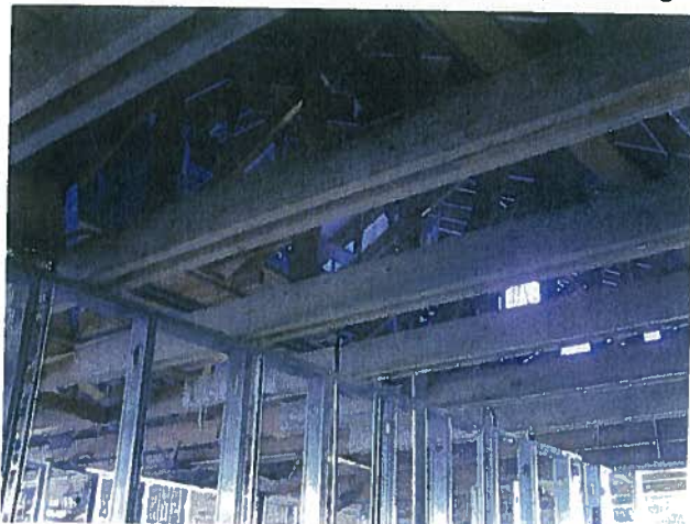
The existing kitchen roof trusses were braced with the addition of new 2" x 6" boards.
