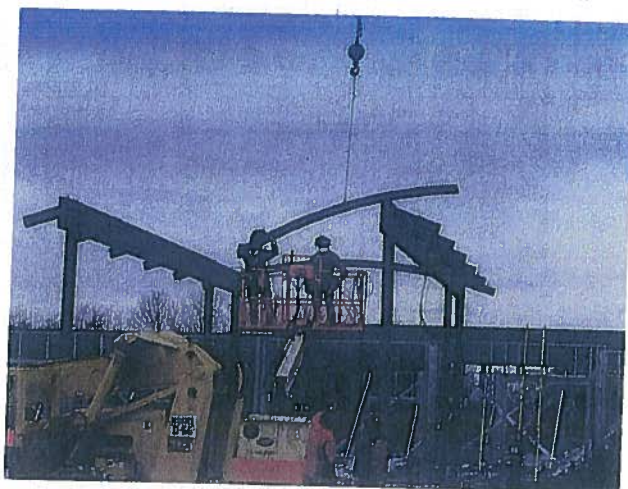
The crane set the arched main canopy support beams in place.
