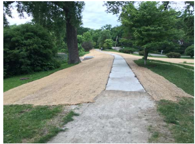
Protective Cap / Sidewalk on Top of Dam and Area Restoration
