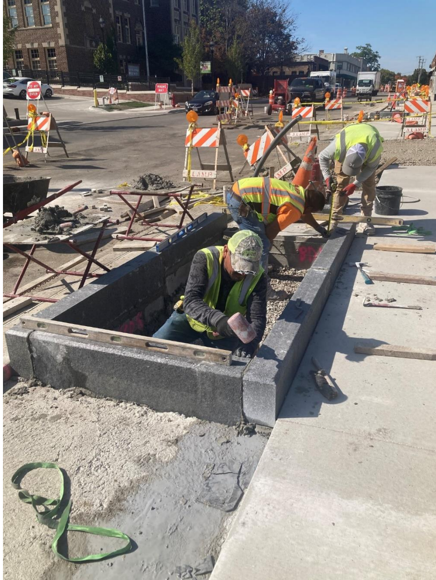
Installation of Granite Curbs on Duane Street – October 6, 2022
