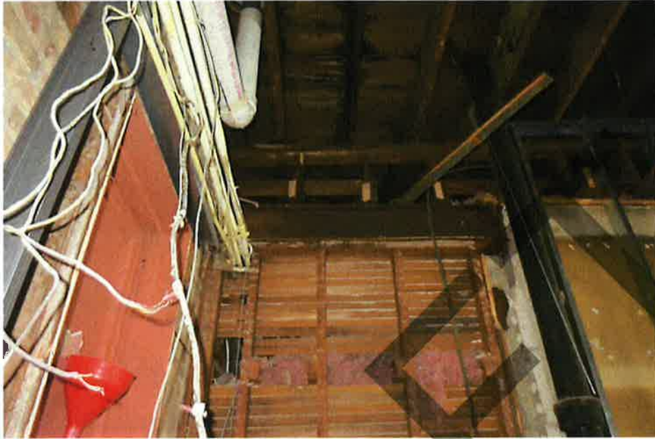
Photo 4: Existing steel beam supporting the roof at the west side.
