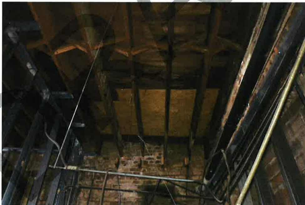
Photo 3: Existing roof framing in 507 Pennsylvania Ave. Joists are 2x12's spaced at 16 inches on center and span approximately 23'-6". Joists bear on CMU wall to the east and a steel beam to the west side.
