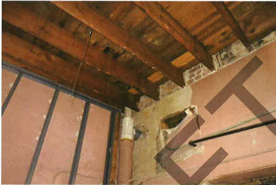
Photo 2: Inside 509 Pennsylvania, the roof is framed with 2x10 joists spanning approximately 16 feet. Joists frame into CMU wall that currently separates the two stores.
