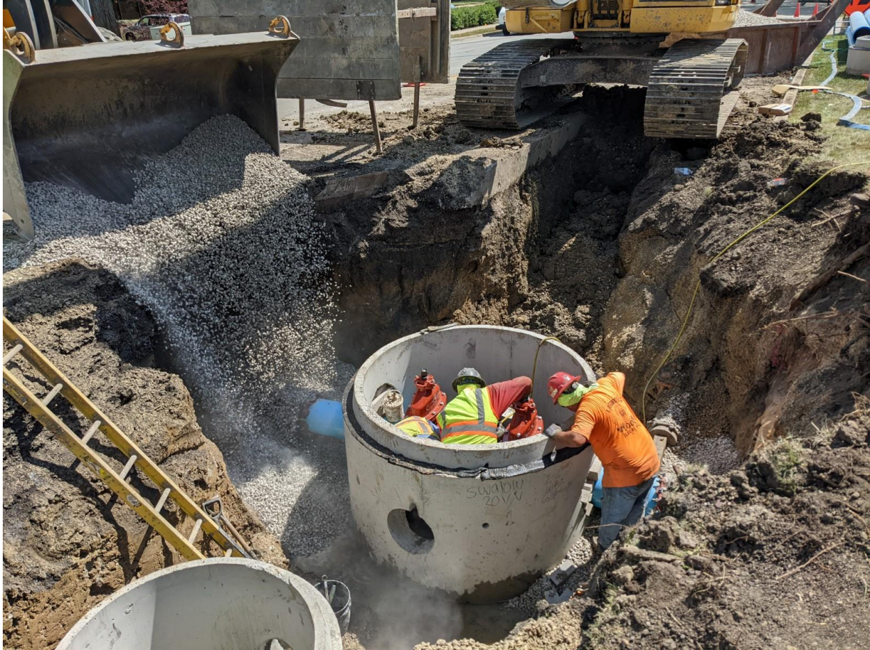
Installation of a valve vault containing a 12" by 12" cross and two 12" gate valves at Park Boulevard and Taft Avenue August 17, 2022
