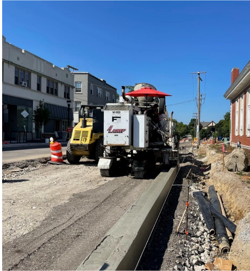
Slip forming of concrete curb & gutter along north side of Duane Street immediately west of Main Street (picture faces west) September 8, 2022
