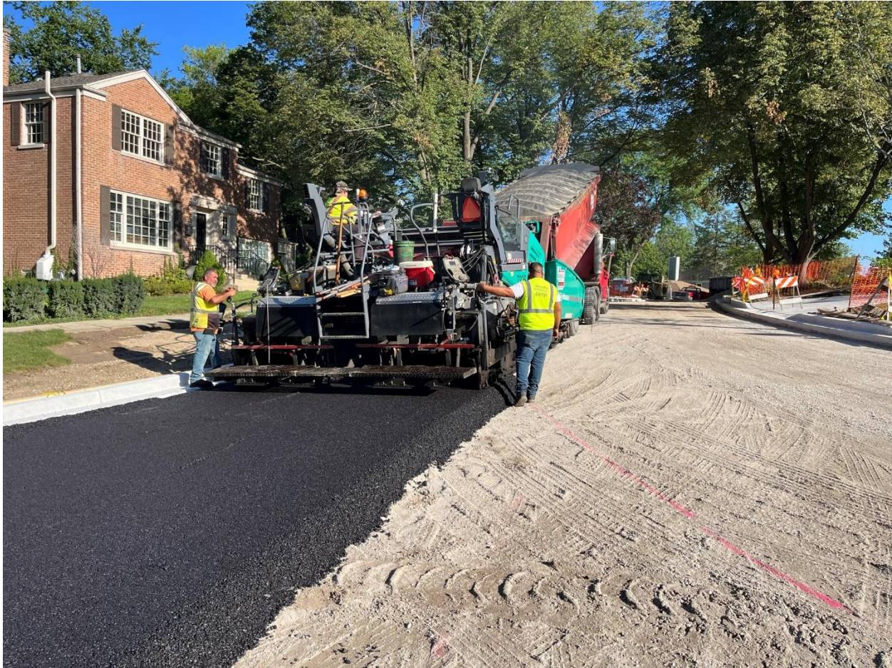
Asphalt Roadway Base Paving on Sawyer Avenue at Windsor Avenue (picture faces north) September 8, 2022
