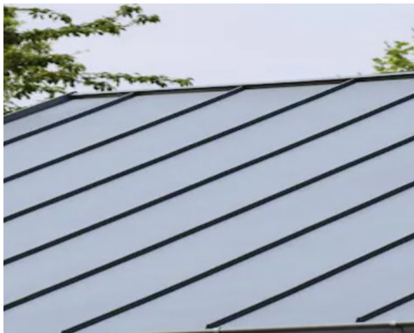
STANDING SEAM ROOF - LIGHT GREY
