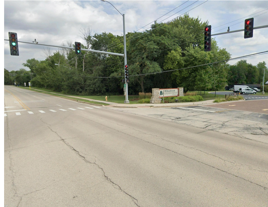
PHOTO 1 - VIEW ALONG PARK AVE
