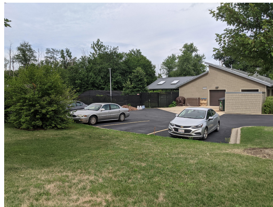
PHOTO 3 - EXISTING ENCLOSURES AND PROPAGATION BUILDING
