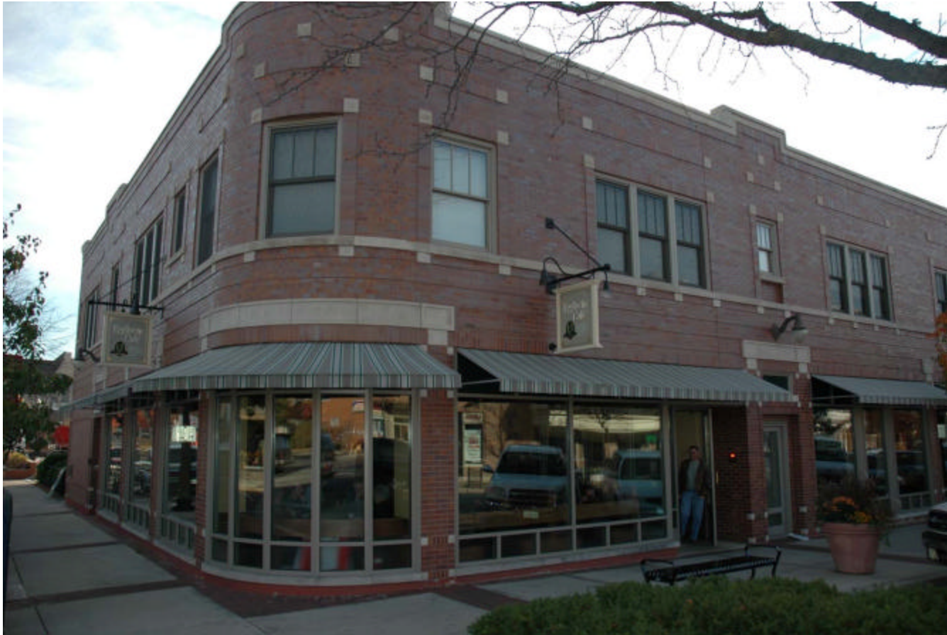
Façade Restoration – Wesley and Hale, Downtown Wheaton
