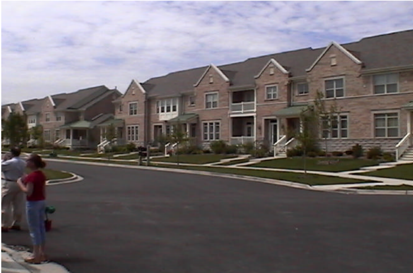
Glenview Naval Air Station Redevelopment – Glenview
