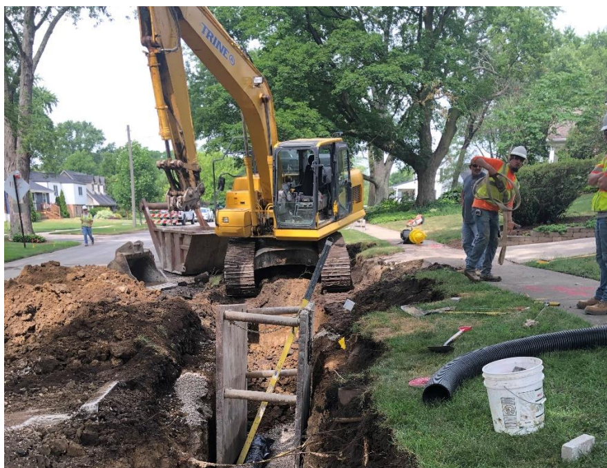
Water Main Installation on Sawyer Avenue
