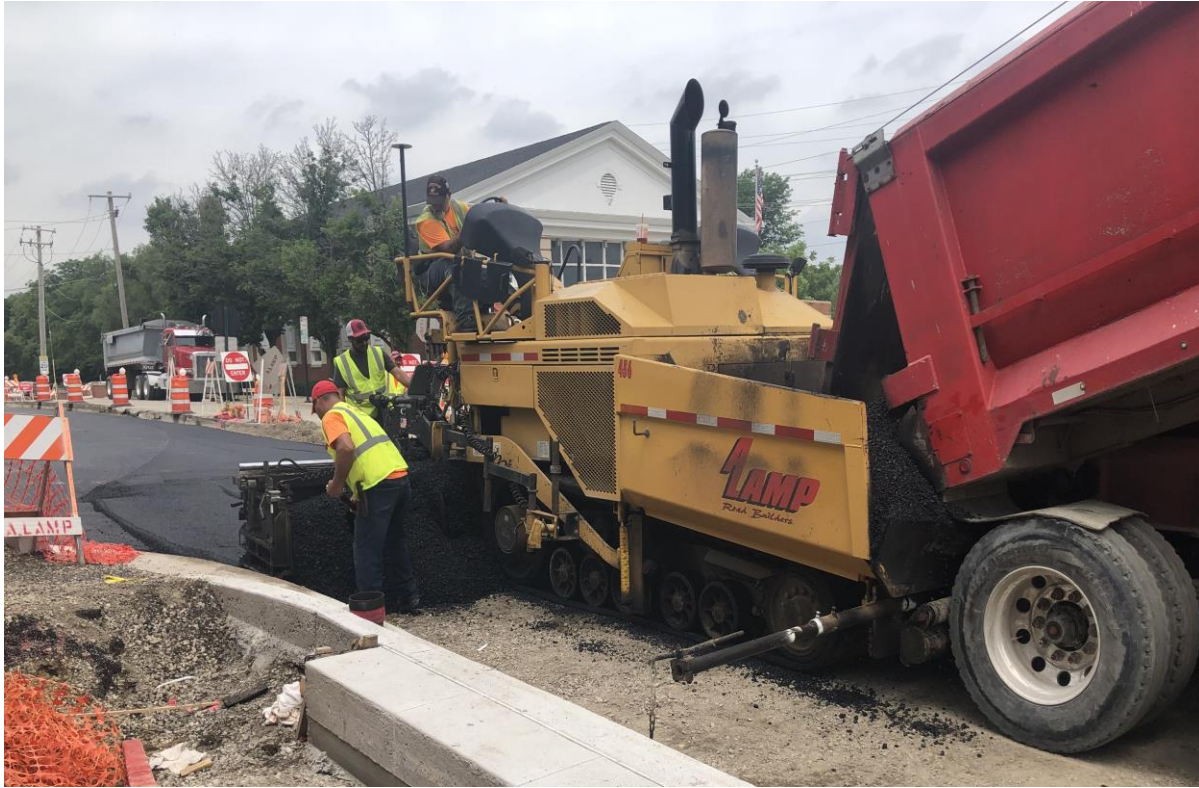
Paving of asphalt binder on Duane Street at Main Street – July 7, 2022
