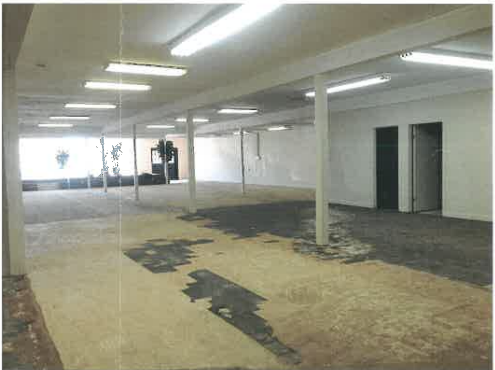
Interior Photograph of Space to be Divided
