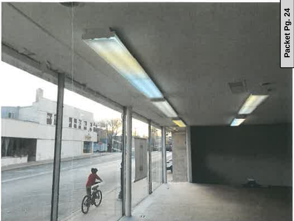
Interior Photograph of Existing Storefront
