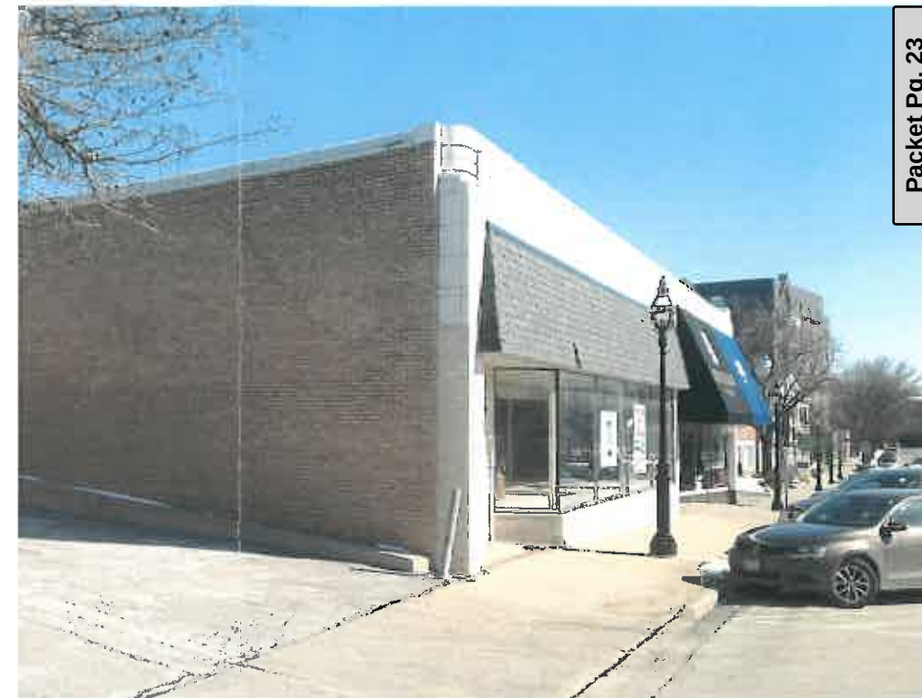
Exterior Photograph from Southwest
