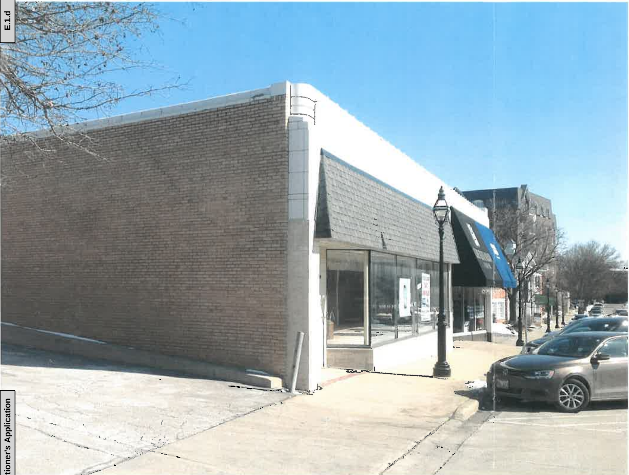
Exterior Photograph of 530-534 Pennsylvania
