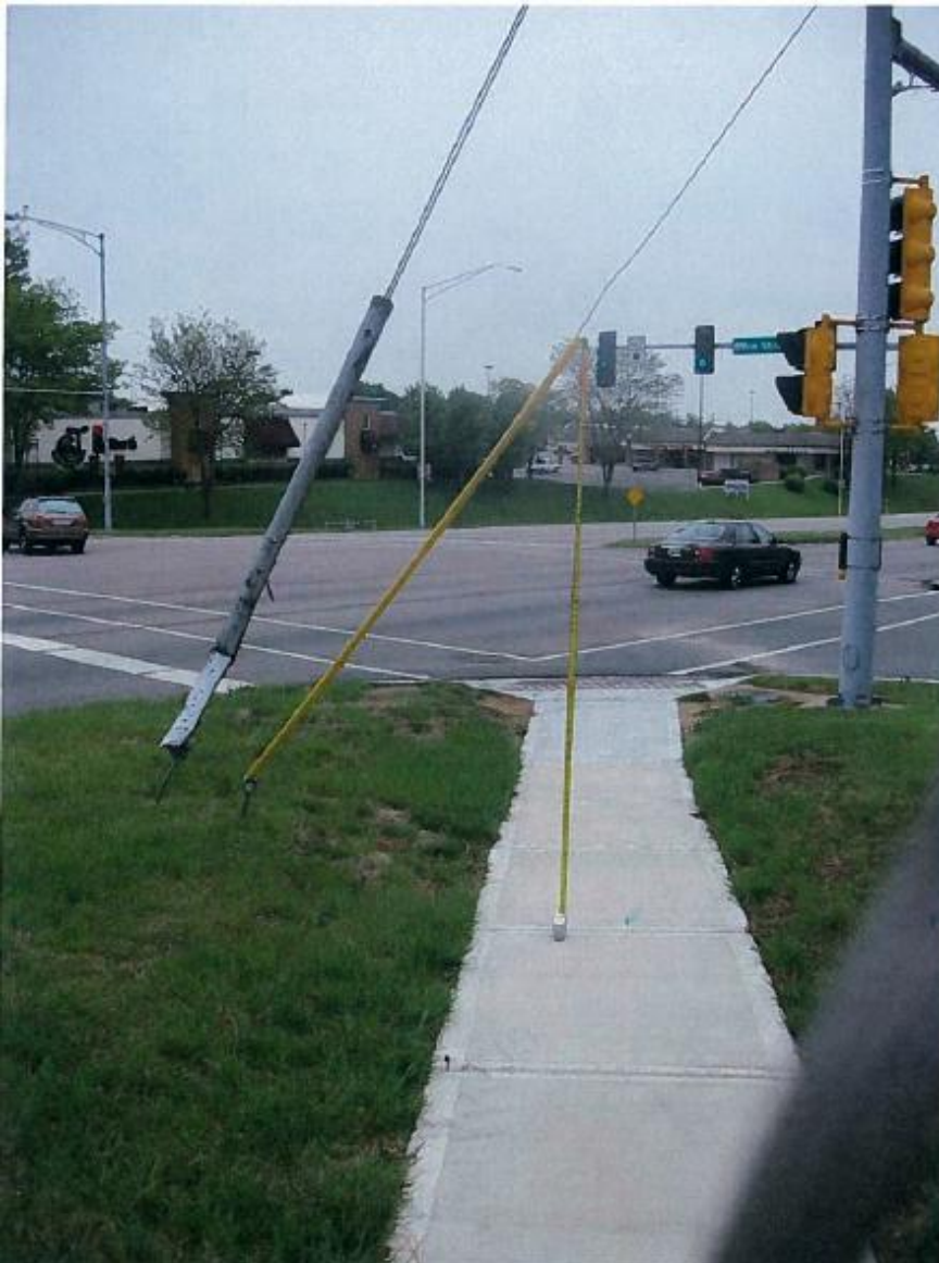
Figure 8 – Protruding Objects (Guy wire is 76" above walk)
