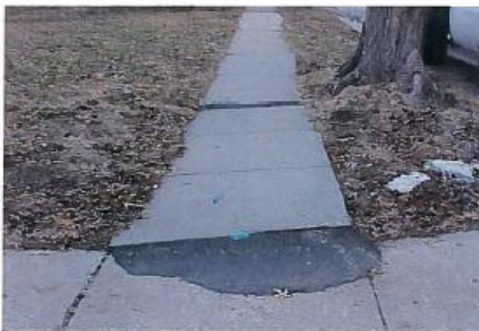
Figure 3P – Patched Fault
