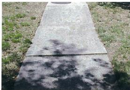
Figure 3L – Faulting 1/2-1"
