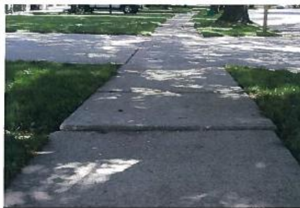
Figure 3M – Faulting 1-2"
