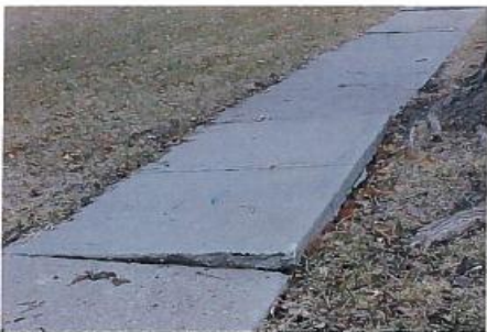
Figure 3H – Faulting >2"
