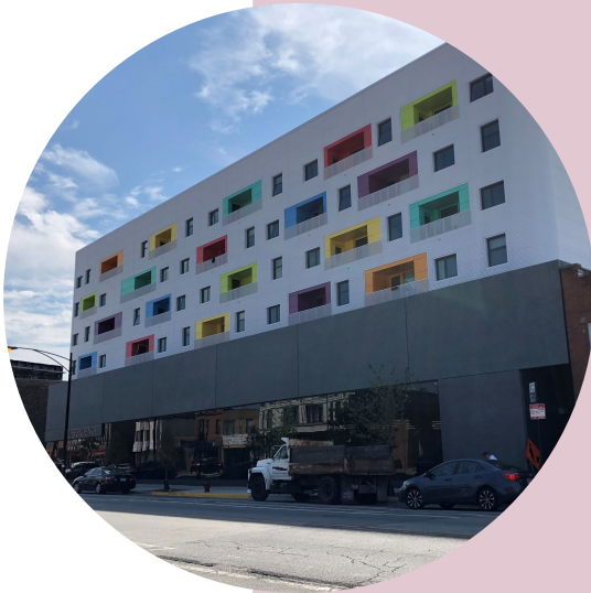
Photo: Independence Apartments
