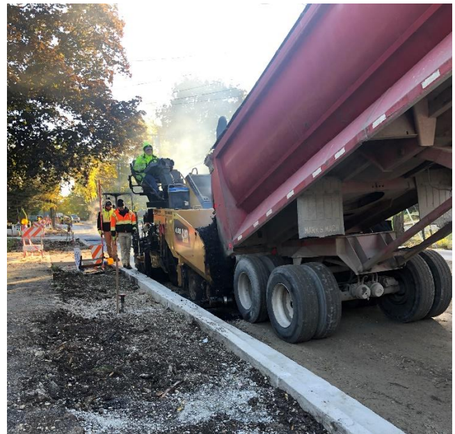
Roadway Asphalt Base Course Paving On Center Street
