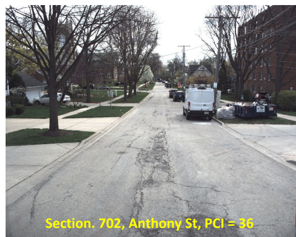
Figure 7. Sample pavement images with different PCI values ('Good' - 'Serious').
