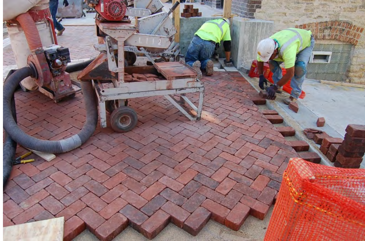
River St, Batavia during construction
