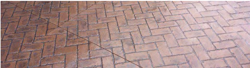
Stamped Concrete: herringbone pattern
