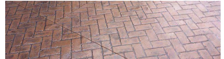
Stamped Concrete: Herringbone Pattern
