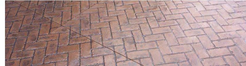
Stamped Concrete: Herringbone Pattern
