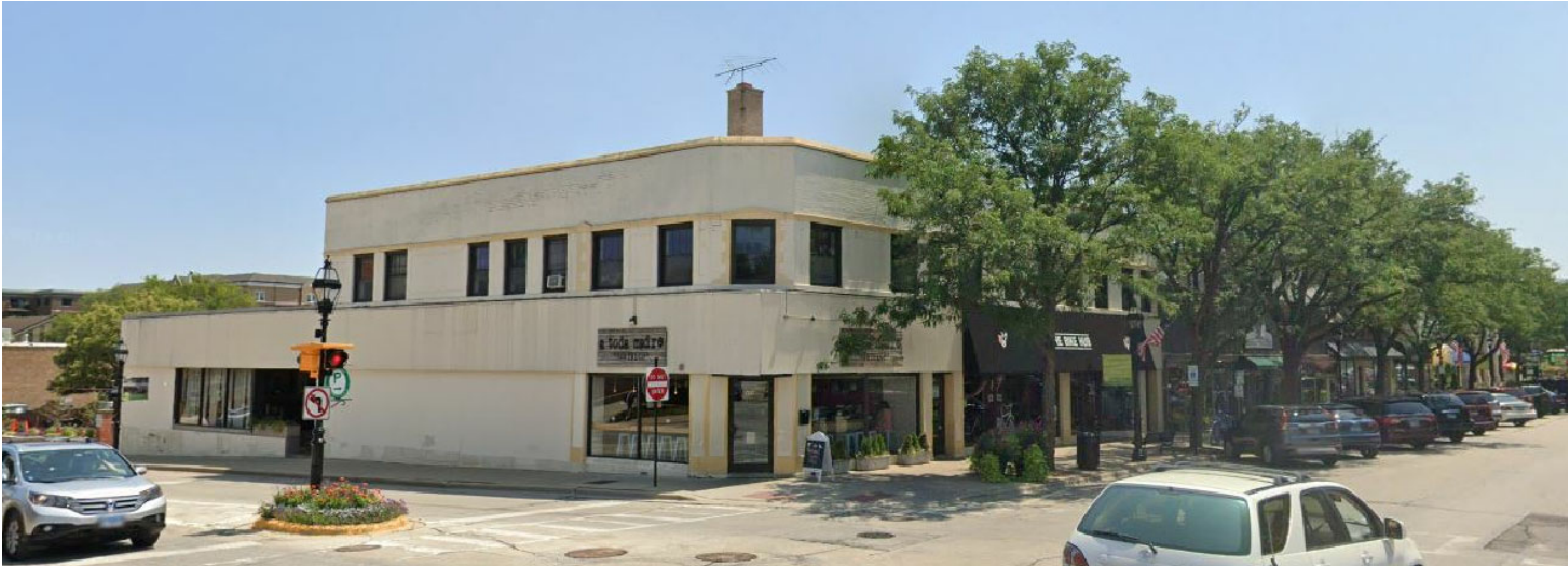
EXISTING VIEW LOOKING SOUTHEAST
