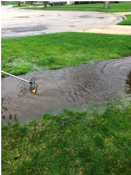
Sidewalk Drainage Issue at 1022 Shady Ln (request & photo from resident)
