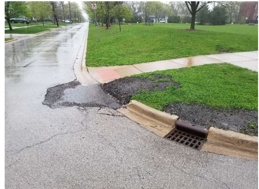
Utility Dig at intersection of Turner Ave & Glenwood Ave
