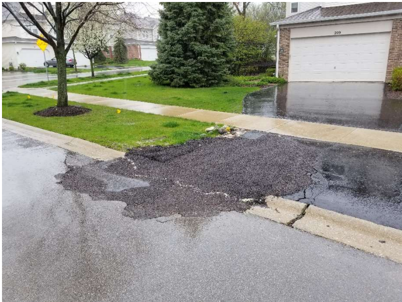
Utility Dig at 209 Tanglewood Dr
