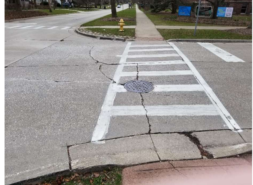
Roadway/Curb at intersection of Main St & Hill Ave
