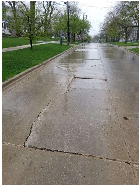
Roadway at 789 Hill Ave
