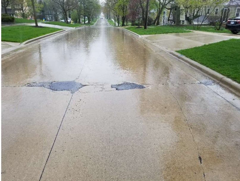
Roadway/Curb at 169 Bryant Ave
