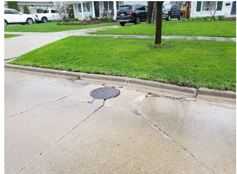
Roadway at 852 Hill Ave
