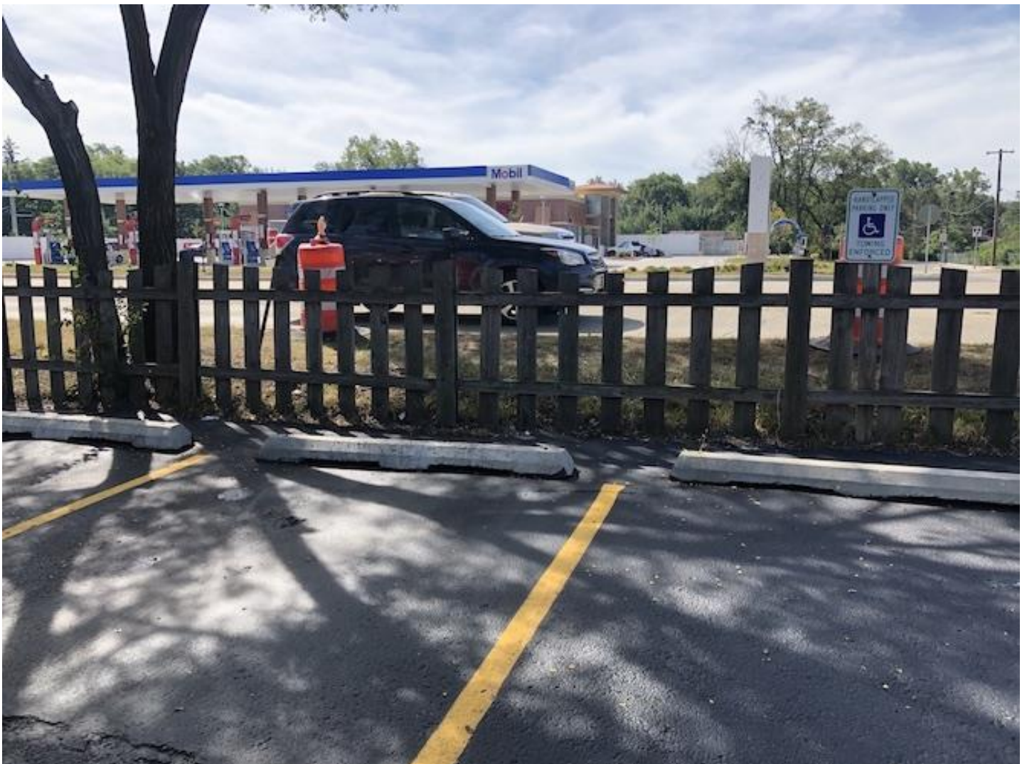
Attachment: 12. Existing Conditions Photos (4608 : Iron Gate Apartments Fence | 11 - 37 Briar Street | Zoning Variation)
