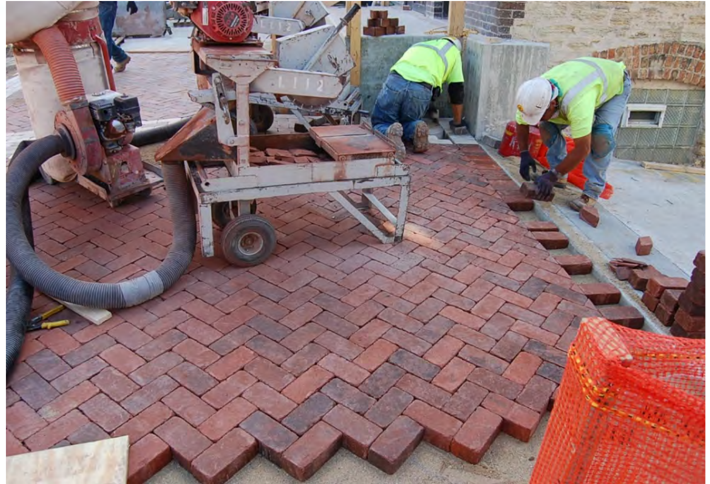
River St, Batavia during construction
