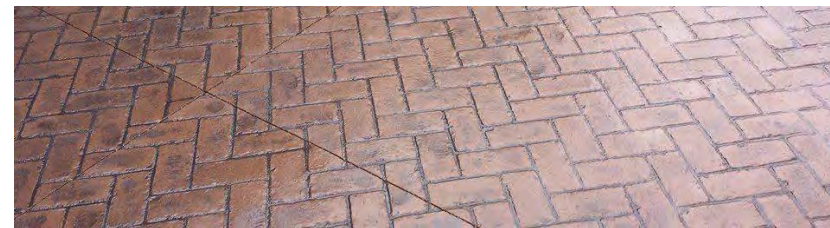
Stamped Concrete: Herringbone Pattern
