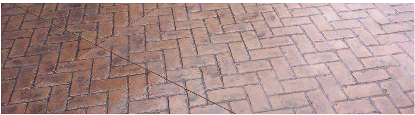
Stamped Concrete: Herringbone Pattern
