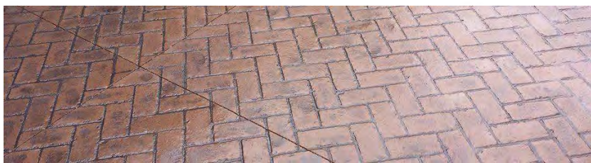
Stamped Concrete: herringbone pattern
