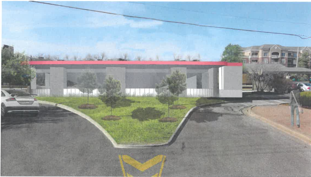
Figure 5 Western Alternative Looking North along Forest Avenue
