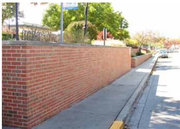
Brick retaining wall
