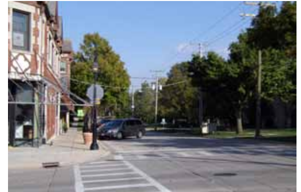
An example of distracting overhead wires
