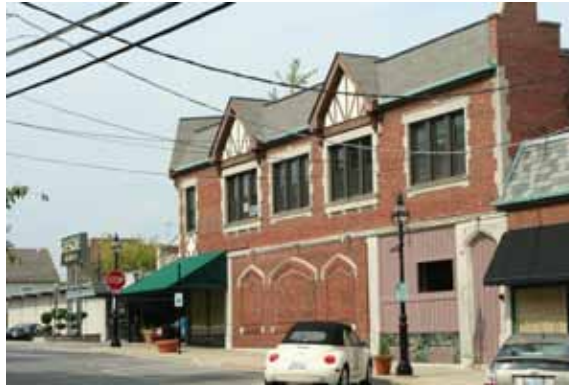
An example of distracting overhead wires
