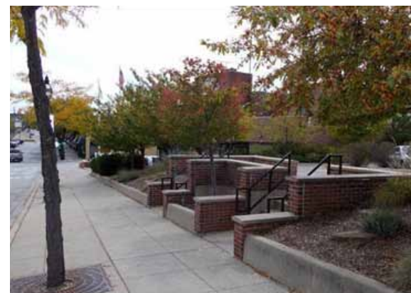
Stepped-back retaining wall
