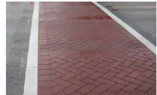
Example of a herringbone brick paver crosswalk
