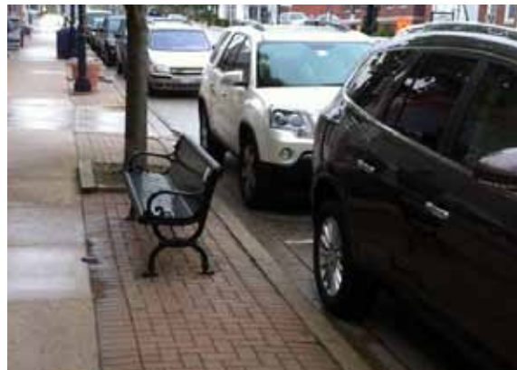
Use of concrete pavers and timbers on Pennsylvania Avenue west of Main Street
