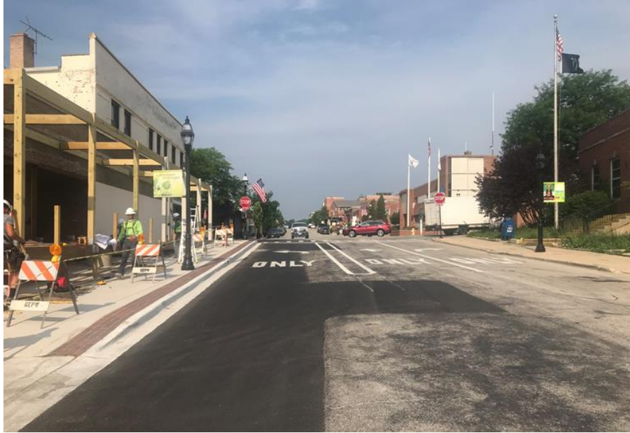
Pennsylvania Ave, looking west at Main St (A Toda Madre dining deck construction in progress)
