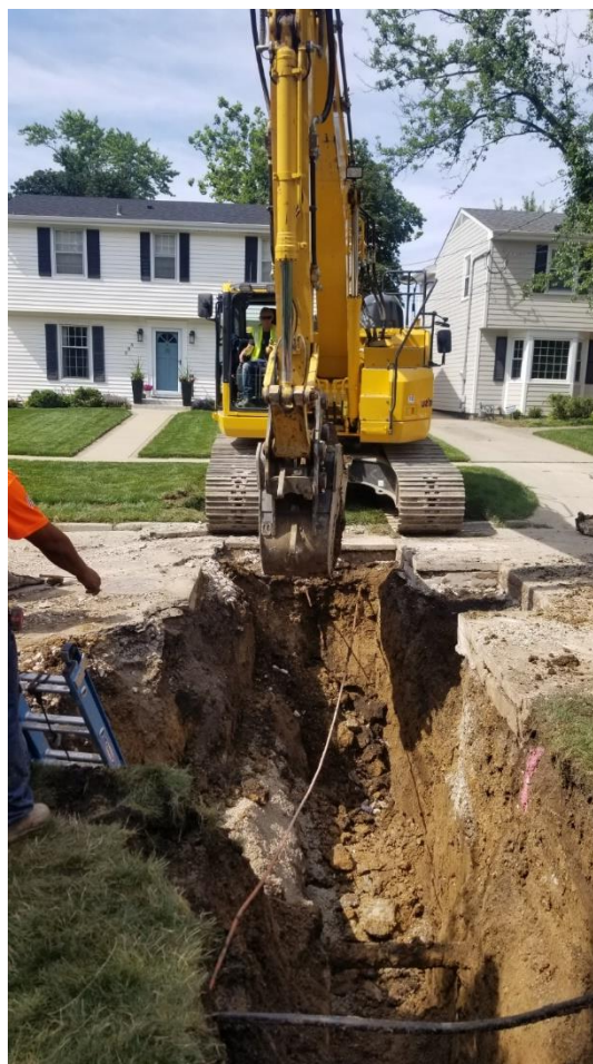
Sewer Service Replacement on Ridgewood Avenue
