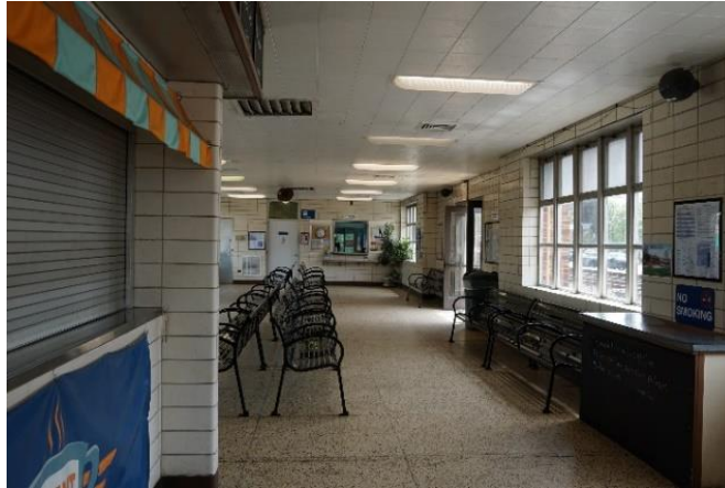
Figure 6: Existing Station Wall Interior – Spine Ceiling, Terrazzo Floors, Structural Tile Wall Surface
