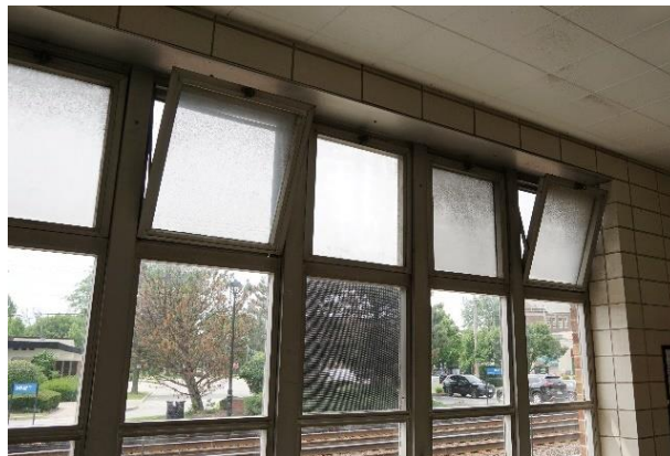
Figure 7: Existing aluminum single pane windows
