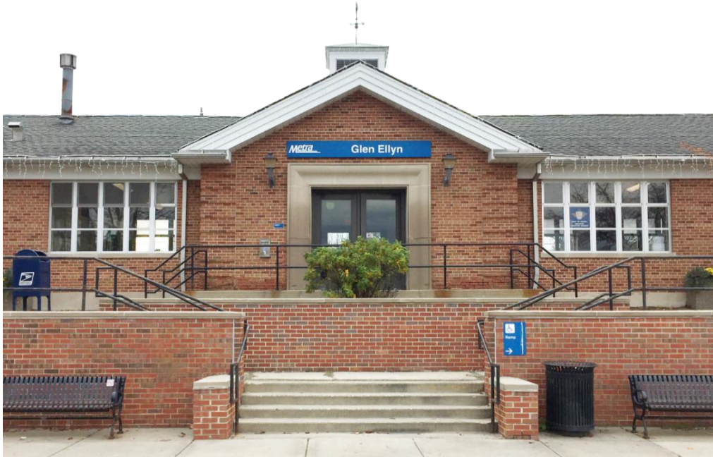
Figure 3: Existing Station Elevation from north looking south
