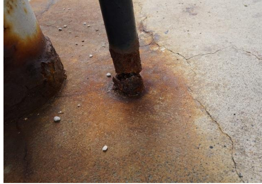
Aging Infrastructure and Structure
