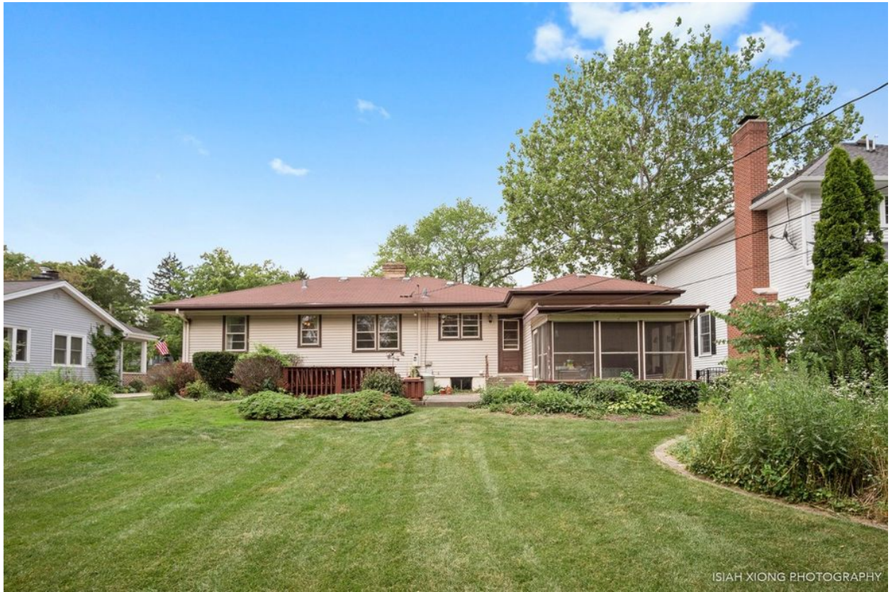
After (back view of house)
