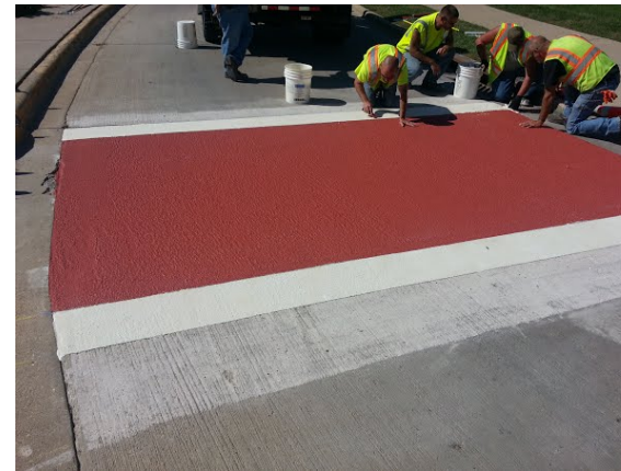
MMA on Concrete
