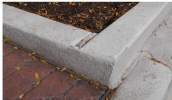
Cast-in-place glitter concrete tree planter curb
