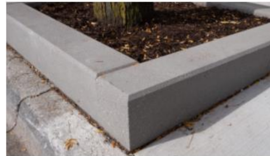
Precast concrete tree planter curb
