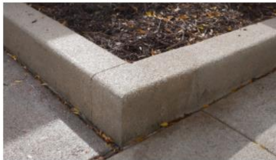
Cast-in-place exposed aggregate tree planter curb
