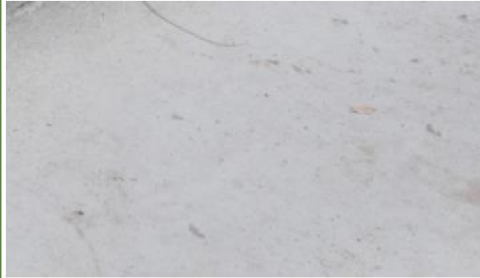
Plain concrete sidewalk
