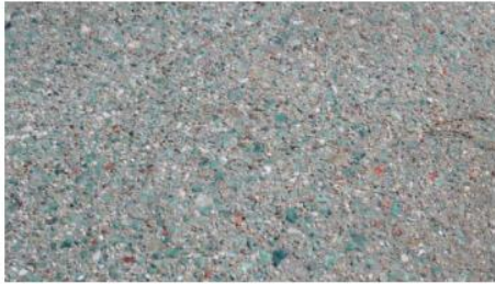
Shamrock green exposed aggregate
