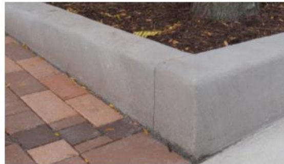
Cast-in-place tree planter curb
