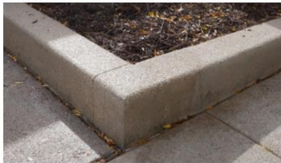
Cast-in-place exposed aggregate tree planter curb
