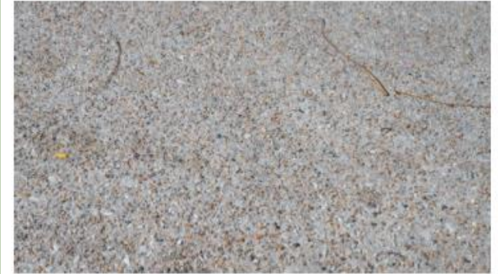
Exposed aggregate concrete sidewalk
