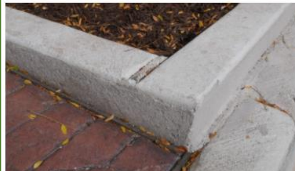
Cast-in-place glitter concrete tree planter curb
