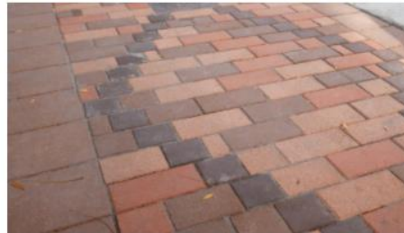
Fired clay brick pavers in a diamond pattern
