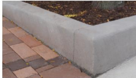
Cast-in-place tree planter curb
