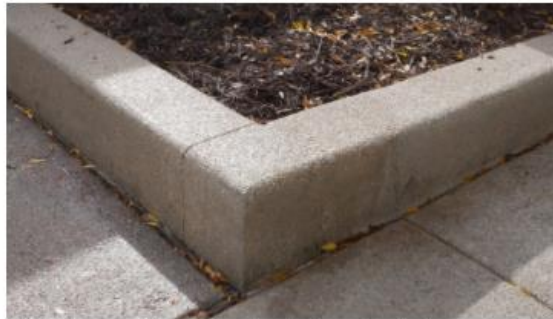
Cast-in-place exposed aggregate tree planter curb
