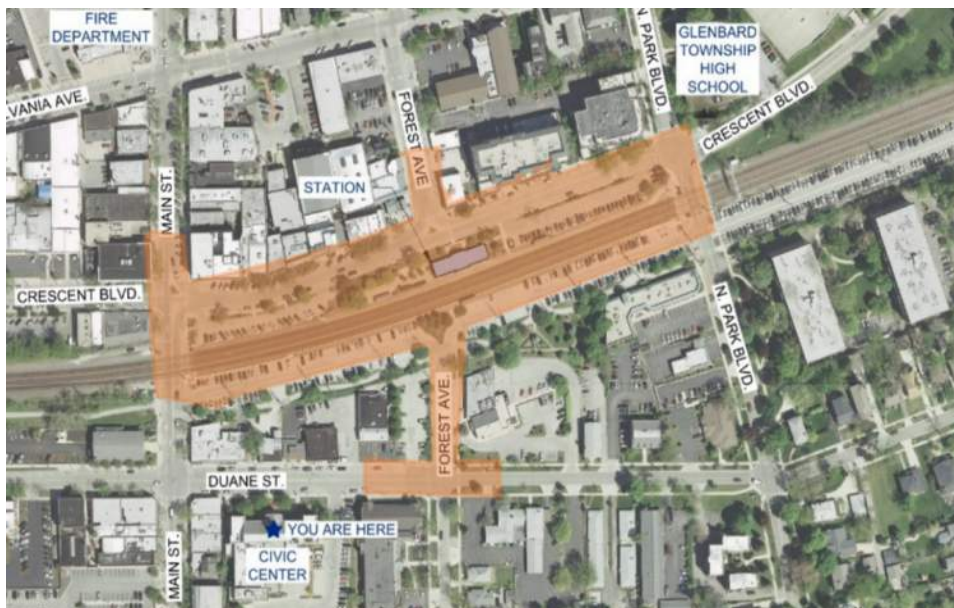
Figure 1: Existing Aerial of the Station and Surrounding Site
