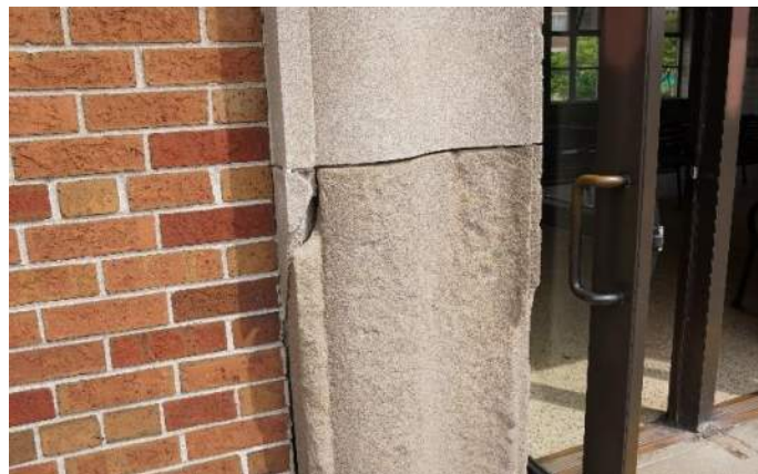
Figure 8: Masonry damage at platform to station entry
