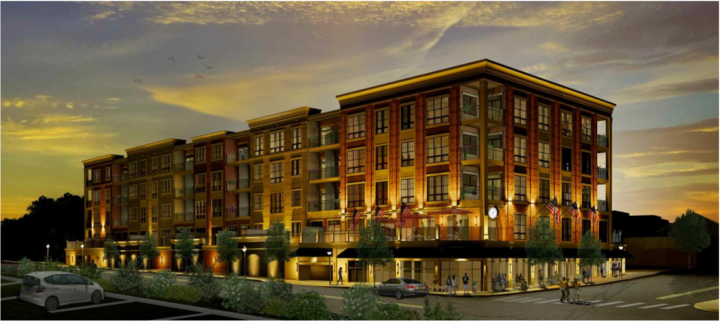
Southeast corner, 9/29/2020 (night)
