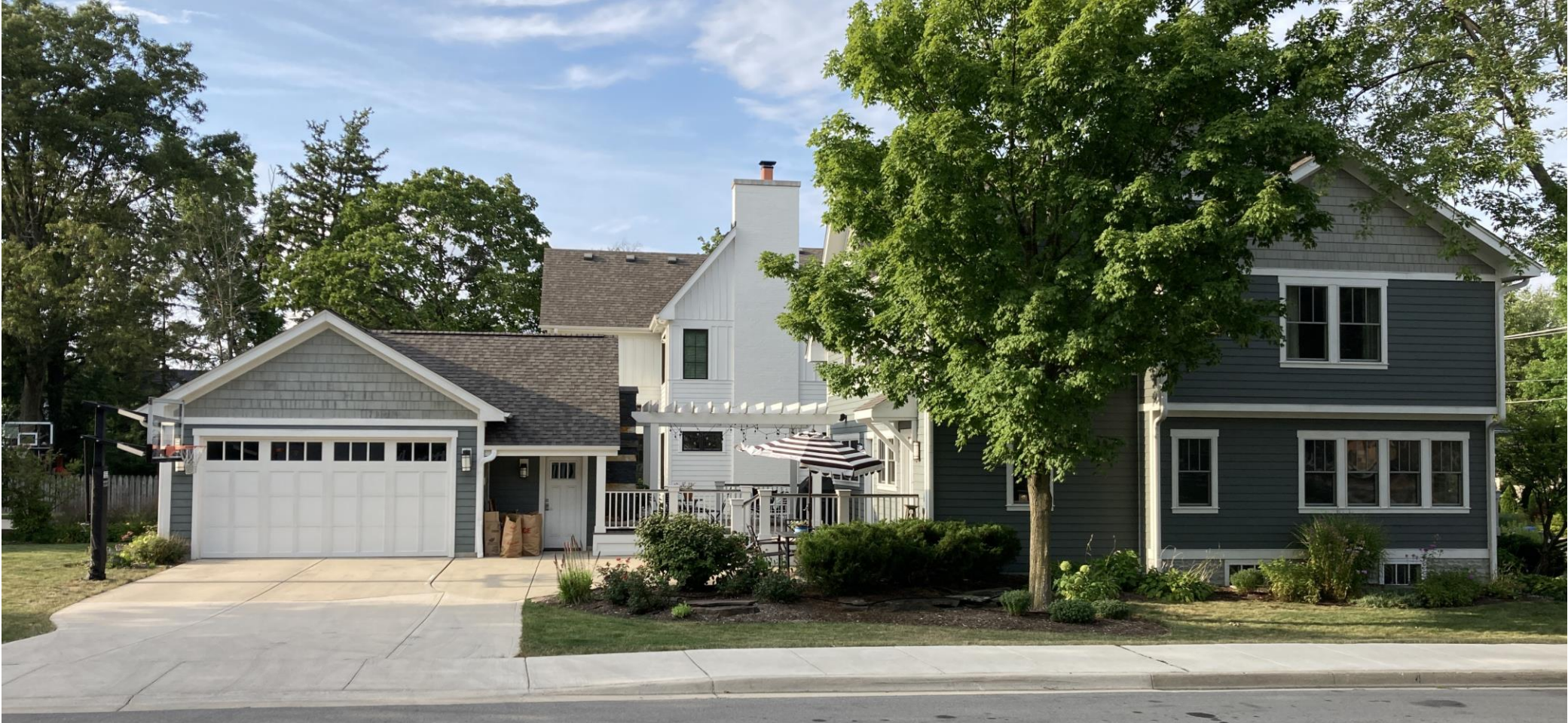
EXISTING SIDE VIEW
