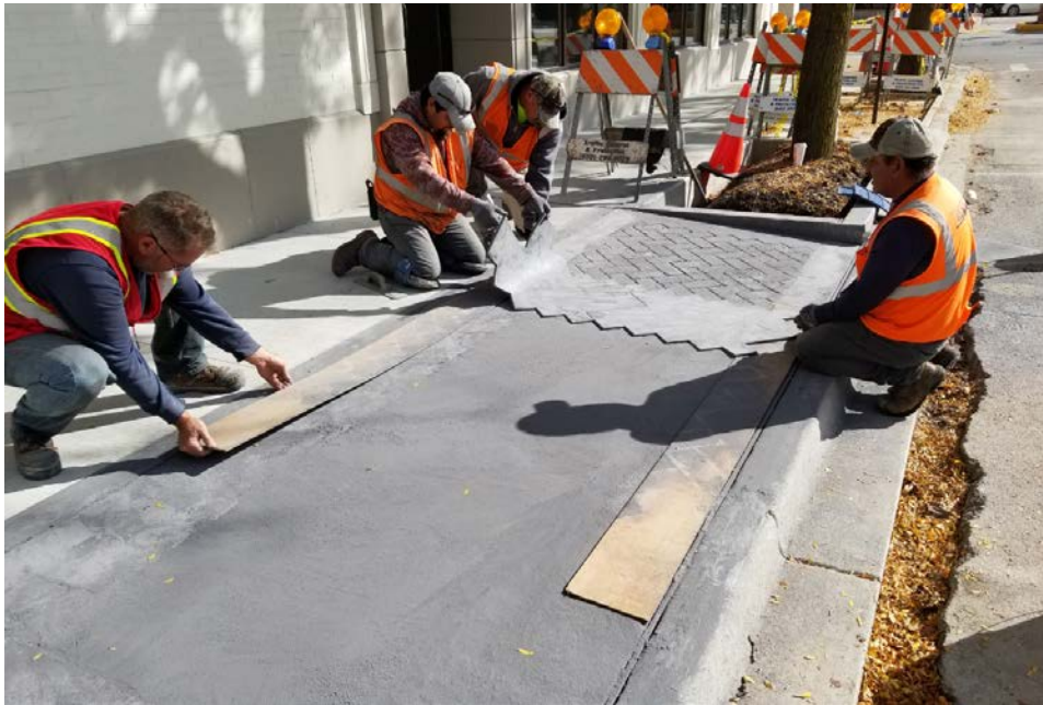
Stamped colored concrete installation on October 1, 2020
