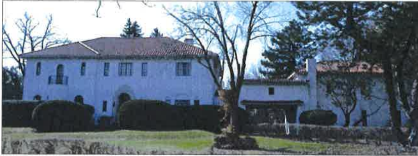
J. K. Marshall House (1930) 583 Hill Avenue
