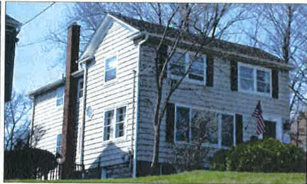
John D. Smith House (1865) 861 Hill Avenue
