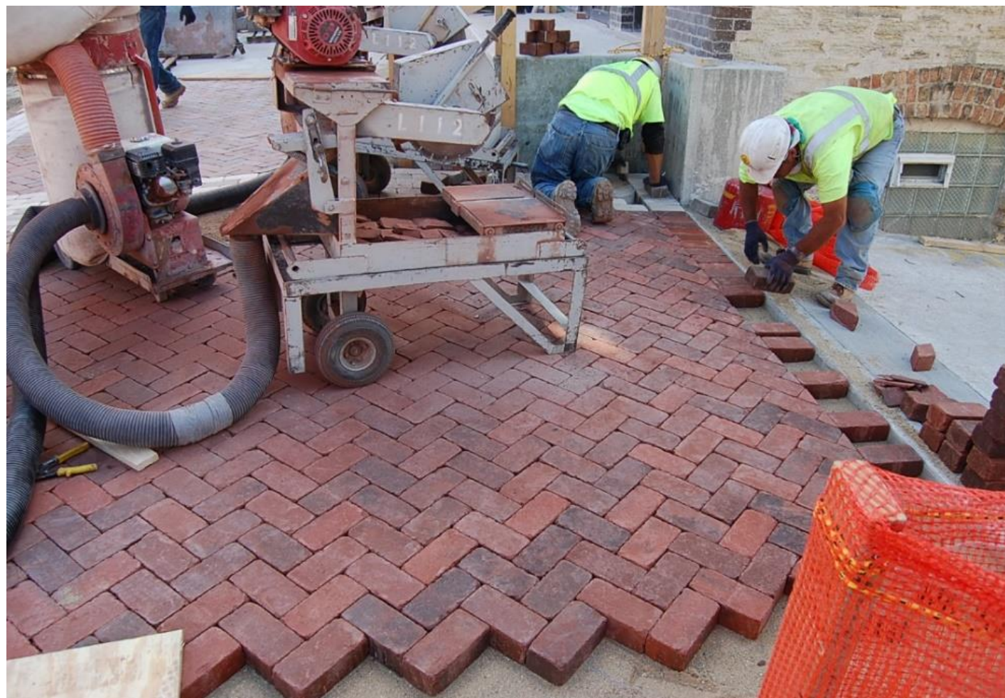
River St, Batavia during construction
