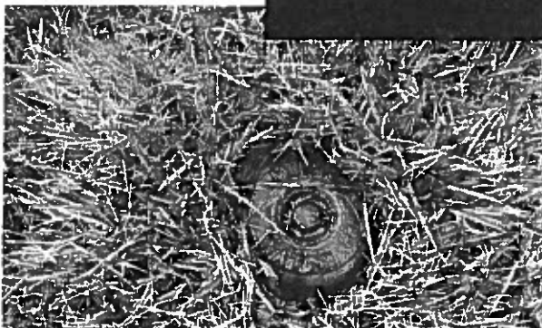
795 Hill Ave. View of second water valve shut off in parkway in front of vacant lot.
