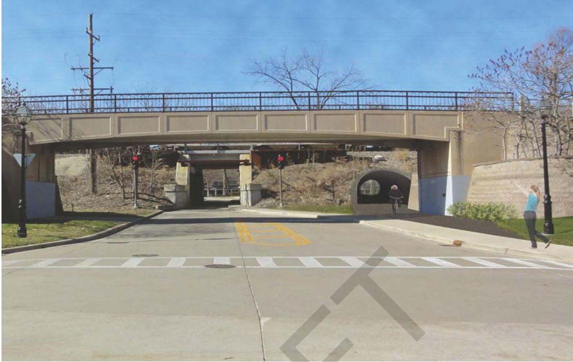
Figure 2 Taylor Avenue Looking North at New Pedestrian Underpass
