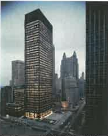
The Seagram Building (1954-8) NYC. Designed by Mies van der Rohe and Philip Johnson.
