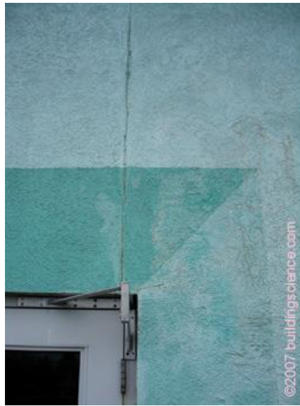
Photograph 2: Cracks in EIFS laminas are often found initially at reveals and at window openings.
