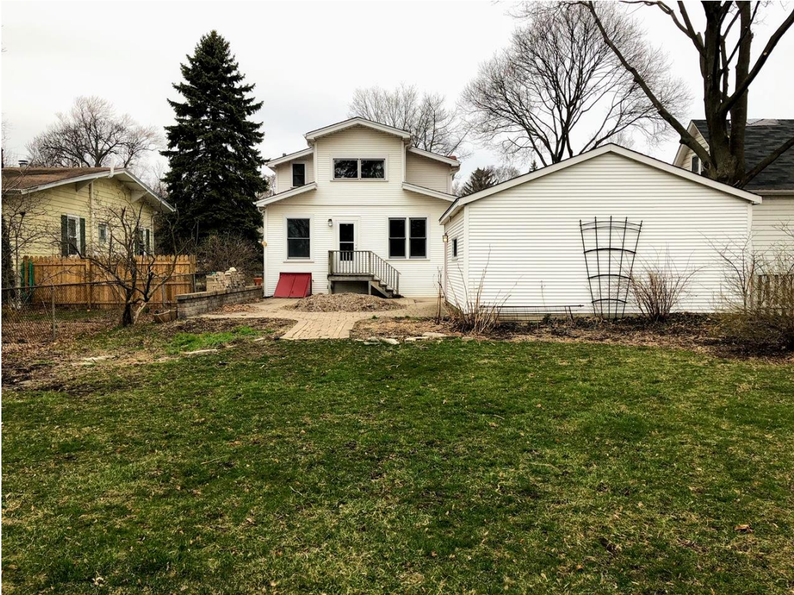
Back of house before
