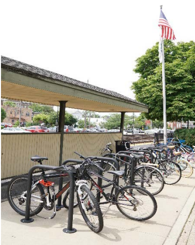
Lean-to at platform, existing bike parking
