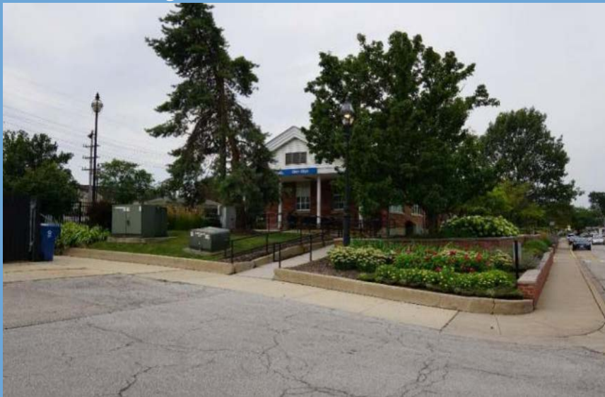
East End of Station Depot
