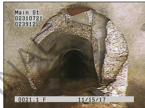
Figure 8 - Break-in Connection at 12" Sewer
