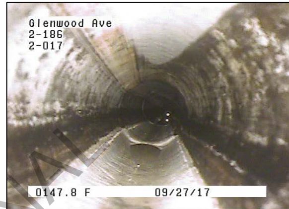
Figure 7 - Evidence of High Water Level
