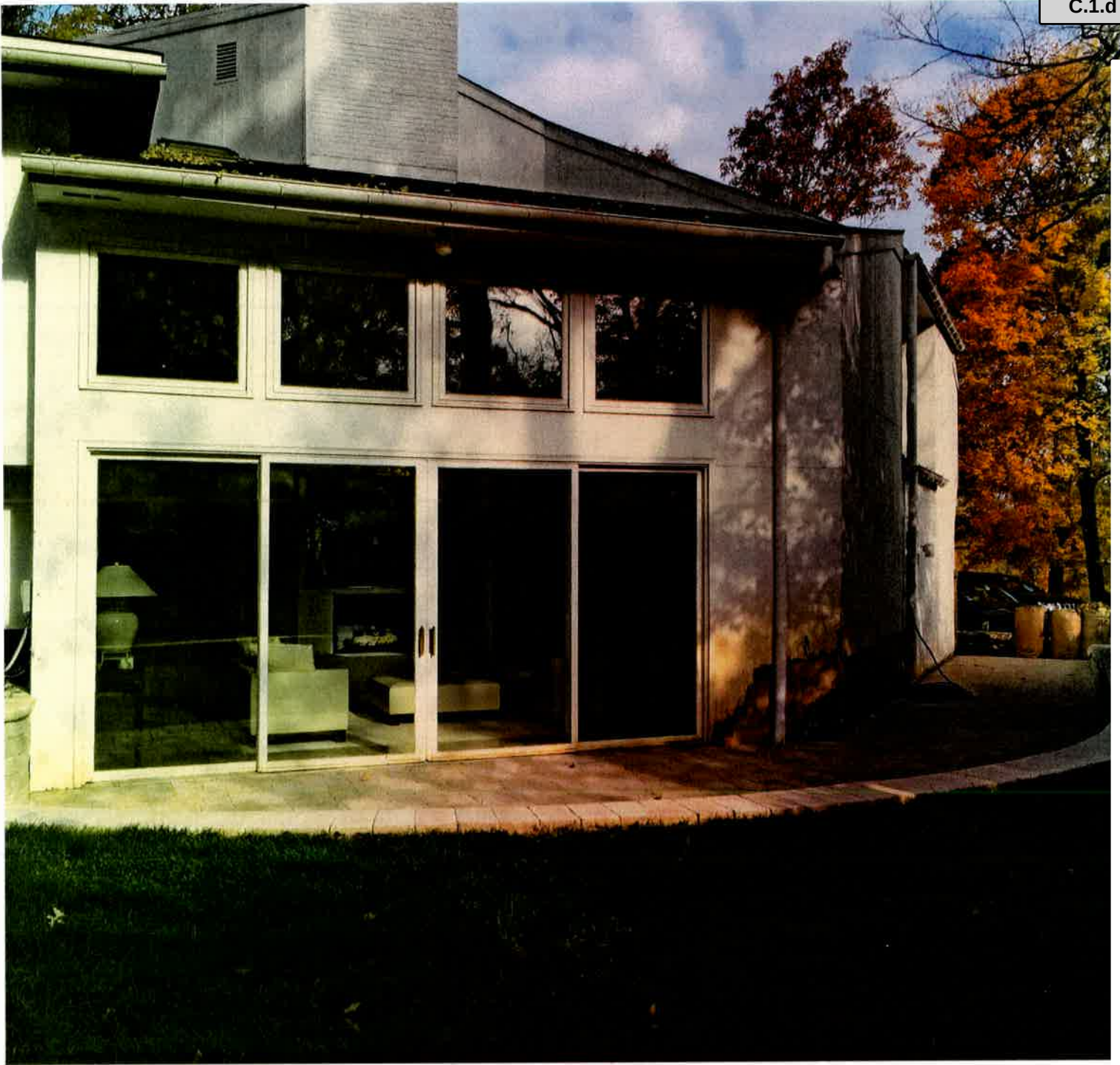
Attachment: Photos - Existing Conditions (3782 : 787 Crescent Blvd. - Accessory Structure Setback & Impervious Surface Setback - CNV)
