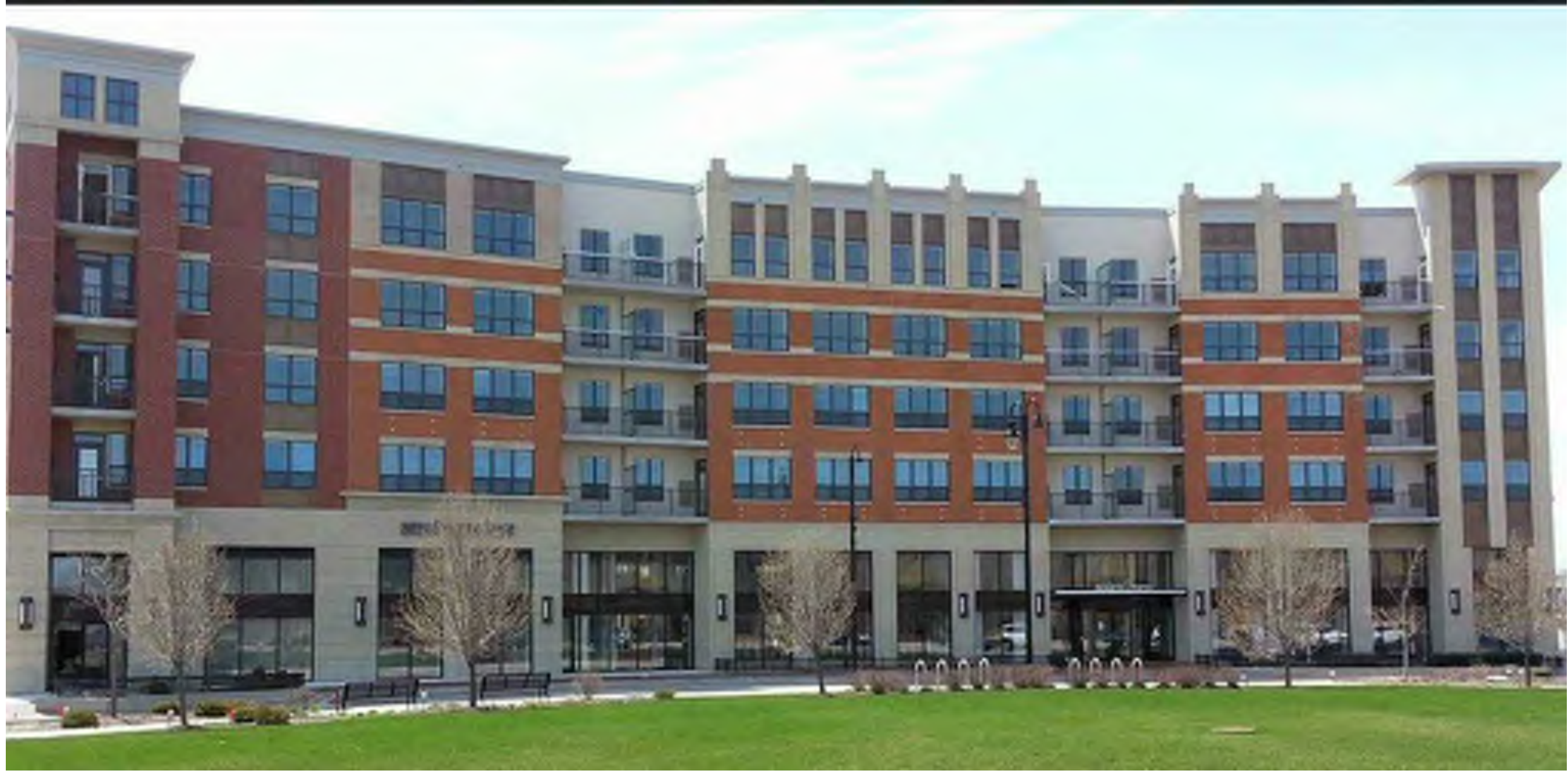
NINETY7FIFTY ON THE PARK, ORLAND PARK, IL
