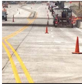
Maintenance of Traffic & Pedestrian Safety
