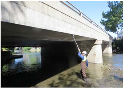
Existing Conditions During Bridge Inspections
