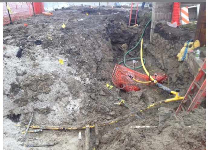
Relocation of gas utilities were required due to conflicting lines on the Rollins Road Gateway.
