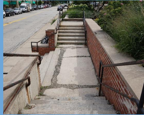
Stairs and Masonry-Aging
