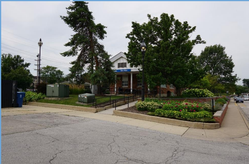
East End of Station Depot
